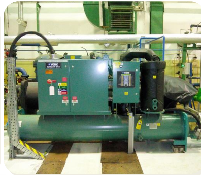
REPLACEMENT OF COOLING UNITS FOR PRODUCTION OF CHILLED WATER FOR HVAC EQUIPMENT
