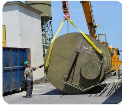
DISMANTLING OF SILOS (CEMENTATION FACILITY)
