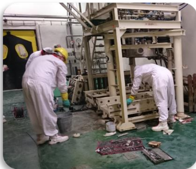
DISMANTLING OF EQUIPMENT (CEMENTATION FACILITY)
