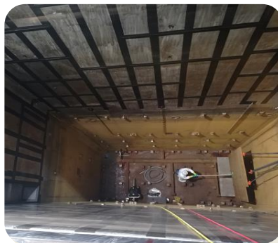
DECONTAMINATION OF SPENT FUEL POOL
