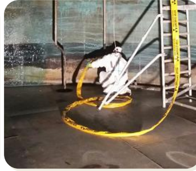
APPLICATION OF DECON-GEL
