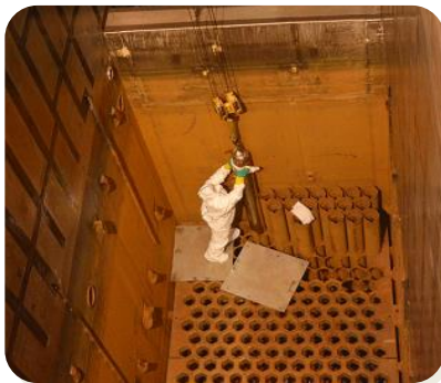
REMOVAL OF HERMETIC CASES FROM SPENT FUEL POOL
