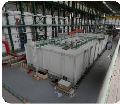
CONSTRUCTION OF DRY CUTTING WORKPLACE IN FORMER TURBINE HALL
