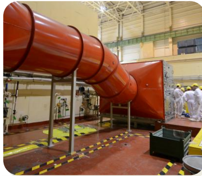
INSTALLATION OF AEROSOL FILTRATION UNIT TO EXHAUST AIR FROM REACTOR HALL
