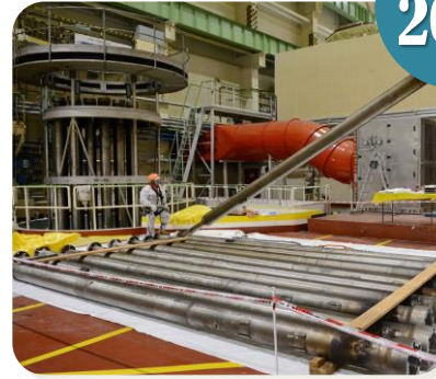
UPPER BLOCK DISMANTLING
