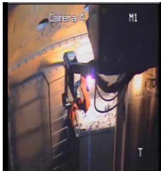
Thermal Column Top Plate Removal
