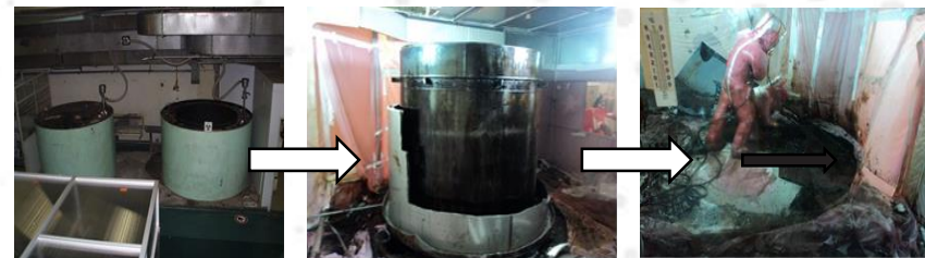
Dismantling of bitumen tanks
