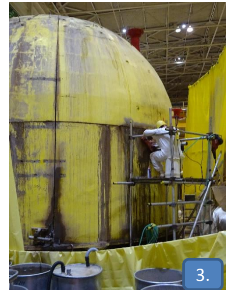
Fragmentation with diamond wire
