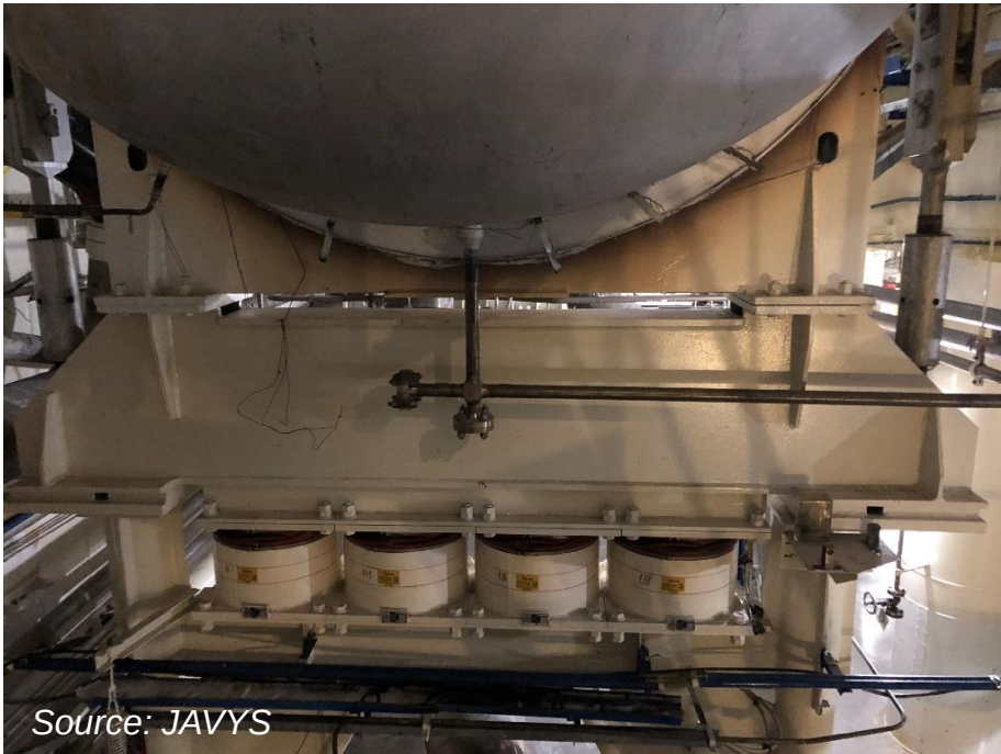
Dismantling of support constructions
