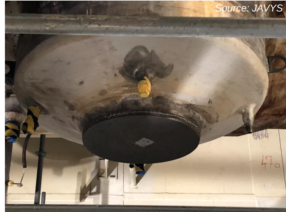
Blinding of SG openings
