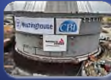
Construction and module assembly
