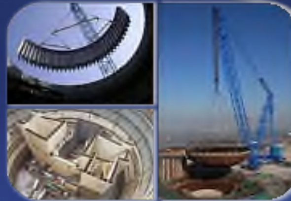
On-site module assembly
