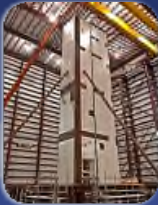
Factory production of modules
